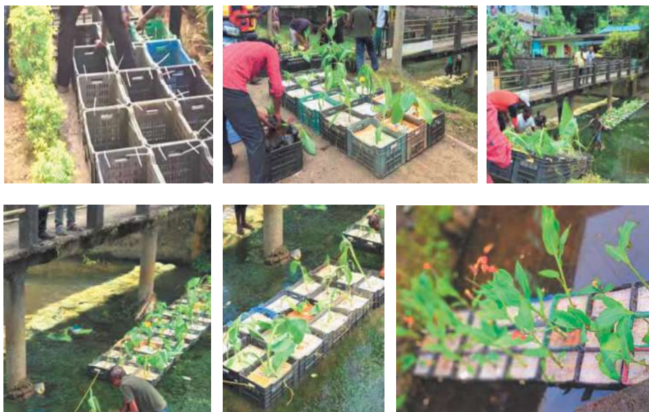
Figure 6 Pilot Project-In-situ N-Treatment system- Corbyn's Cove Drain
