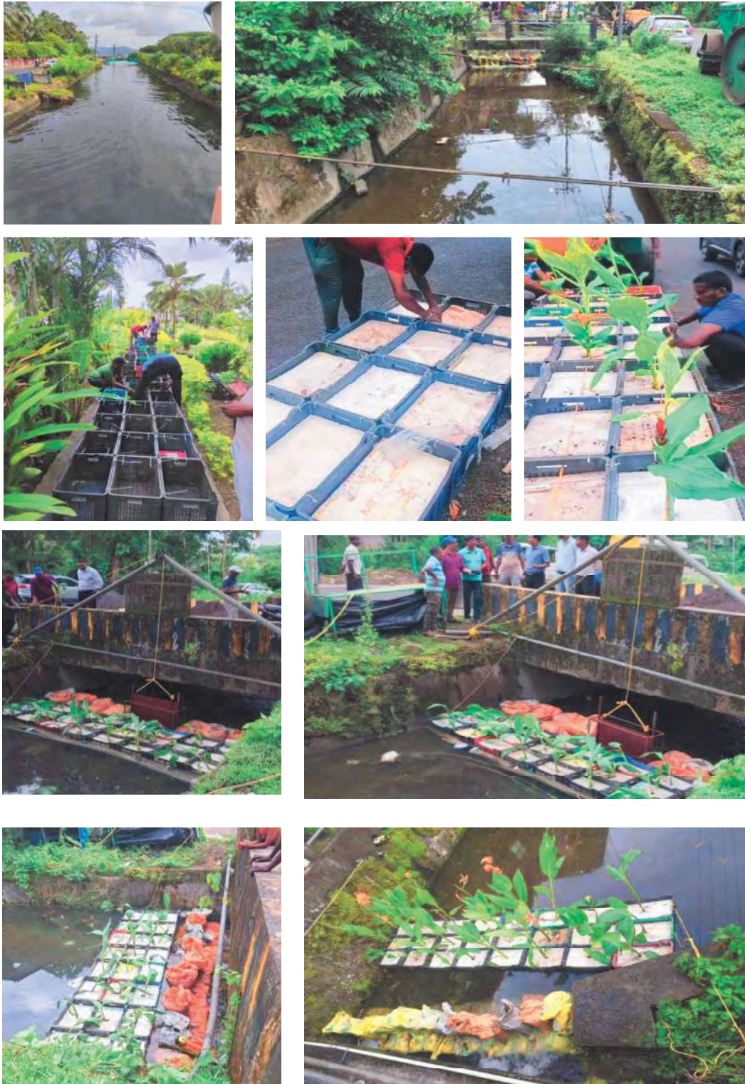
Figure 5 Pilot Project-In-situ N-Treatment system- R.K. Mission Drain
